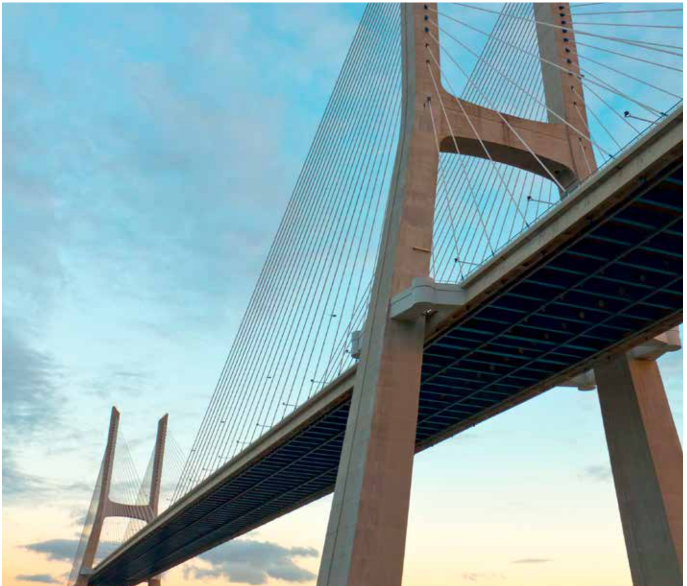
Vasco da Gama Bridge, Lisbon, Portugal
